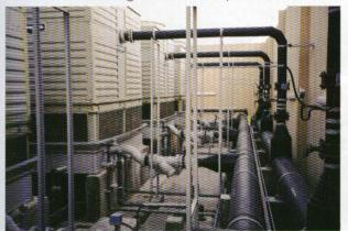
head pressures on the compressors of the water cooled plant, it is envisaged that the overall operating cost saving of the water cooled plant will be in excess of 30% lower than that of the existing phase 1 air cooled plant.
